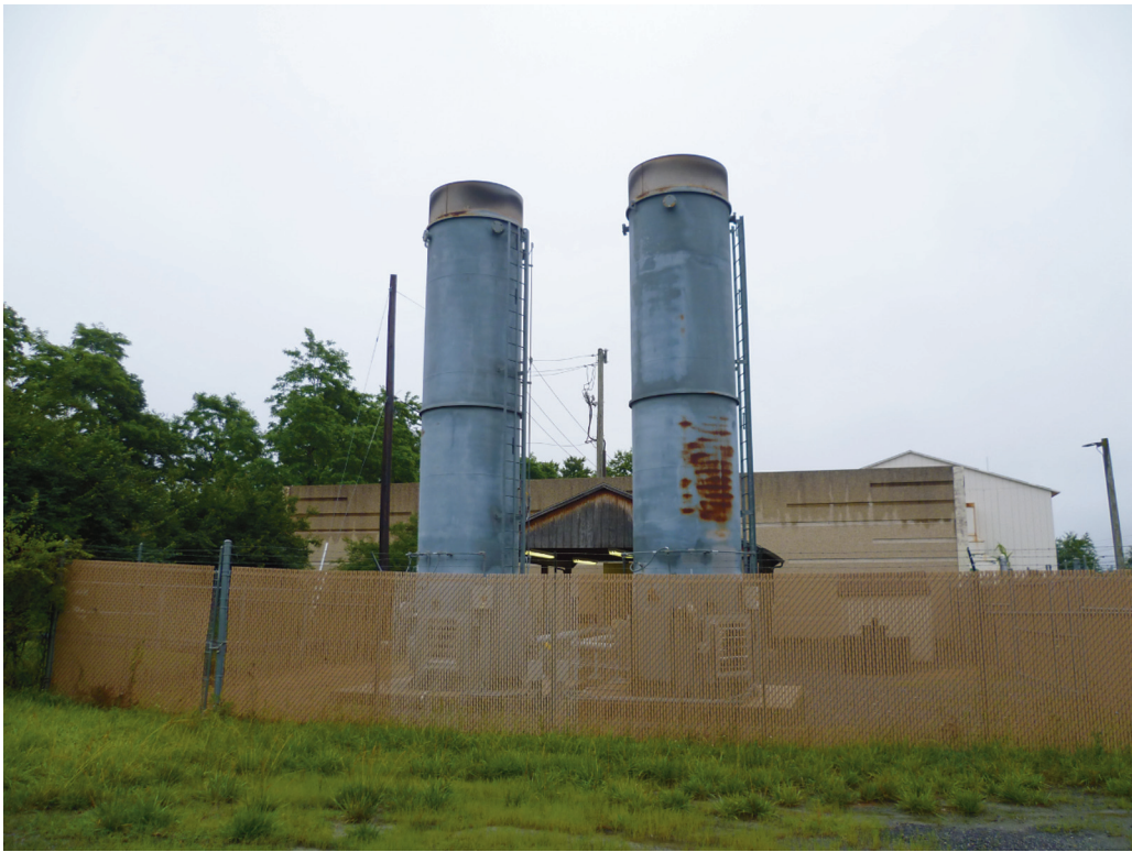
Figure 2 Photograph of the methane flares at the time of the site visit. (Photo by NIOSH.)
