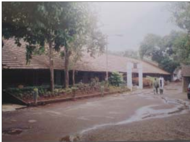
Figure 1: The 'old barracks' which formed the first wards of Dr. A. D. Dias
